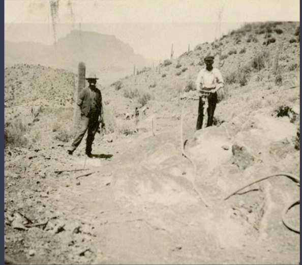
Right: Arizona Historical Society, MSS 130 Charles A. Barrow Collection, 100-0004425: Using an air drill while doing road construction, c. 1920s.
